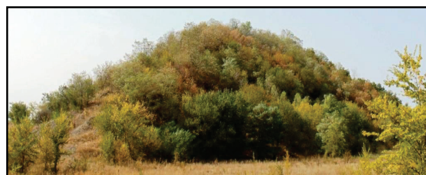
Fig. 19. View of the north-eastern side of waste dump No. 1 in October 2019
